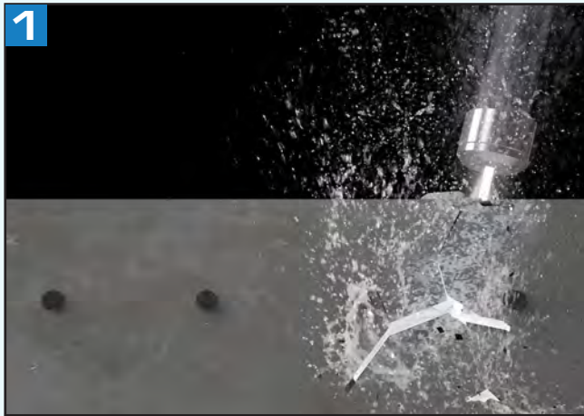
The water jet penetrates existing cavities and cracks.
